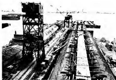
The tunnel sections, each the length of a football field, were towed to this shape-up basin in Fairfield. Here much of the interior work was done, including the laying of the roadway.
